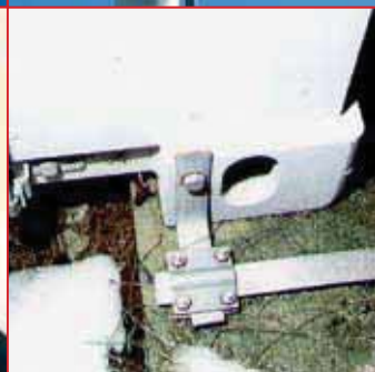
连接于接地系统的屏蔽架 Bonding of a shelter to the earthing system
