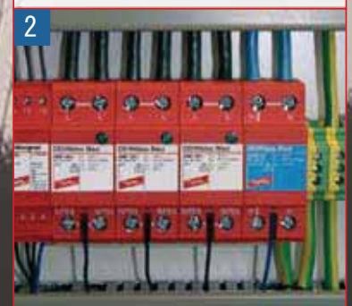
安装在开关柜中的DEHNBloc® Maxi 和 DEHNgap Maxi DEHNBloc® Maxi and DEHNgap Maxi in a meter cabinet
