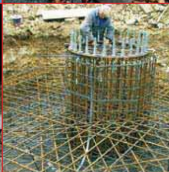
带接地棒的地基 Foundation with foundation earthing electrode
